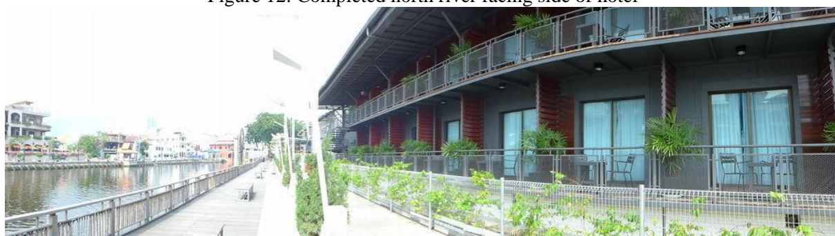
Figure 12: Completed north river facing side of hotel
