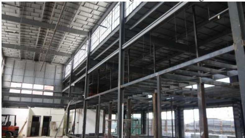
Figure 5: Structural reinforcements to the original structure using I-Beam construction
