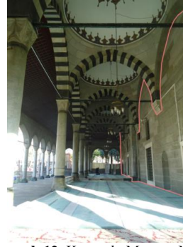
Photograph 12. Kurşunlu Mosque Northern Façade (Merve Hasözhan, 2016)
