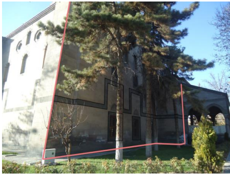
Photograph 13. Kurşunlu Mosque Eastern Façade (Merve Hasözhan, 2016)
