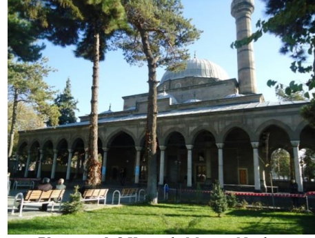
Photograph 8. Kurşunlu Mosque Northern Façade (Hürmet Çopuroğlu, 2016)
